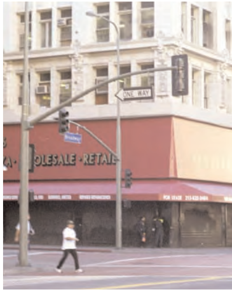
Some building owners have implemented interim solutions such as this awning, which unifies the storefront. In the future, the building owner could restore the transom windows and provide individual awnings for each storefront.
