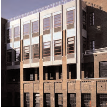
This rooftop addition continues the lines and materials of the original building before transitioning into new materials and forms. This technique creates a more seamless intersection between new and old.
