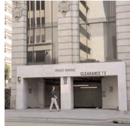
Do not cut new entrances on primary facades where no entrance originally existed.
