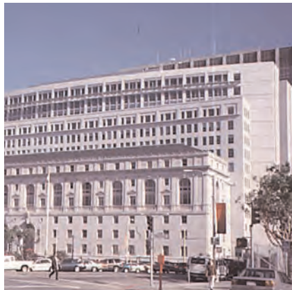
The addition to the State Courts building in San Francisco steps up and back from the original structure. This is a more appropriate approach to a building addition than the project shown above.
