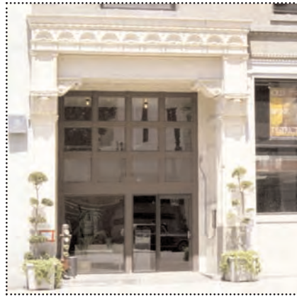
After the entrance was rehabilitated, the security grille was removed, the doors and transom windows were restored, planters were added, and the overall entrance is a much more attractive and inviting space.
