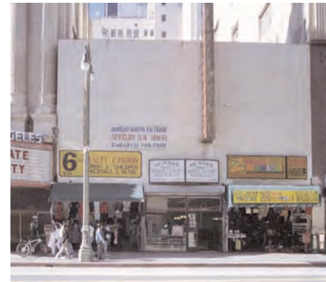
Unfortunately, the Los Angeles Theater’s north storefront has been covered over. Testing, as a first step, may determine if any historic fabric remains. If no material remains, the south storefront could be used to pattern elements and replicate missing features.
