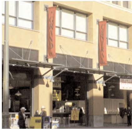
The lightweight quality of the Grand Central Market's awnings complement the simple lines of the building, and create an intermediate zone between the public area of the sidewalk and the private area of the Market.
