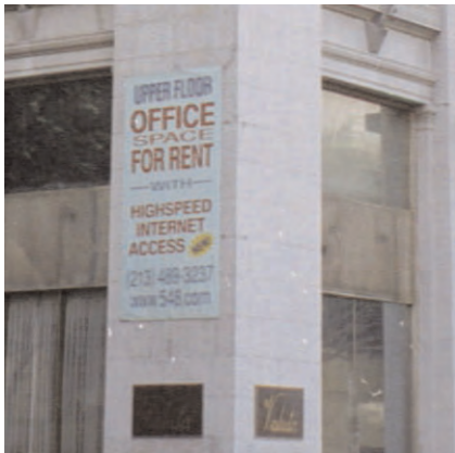
Use of computers has changed the way buildings are wired. Consideration of this aspect of daily life is now an important part of system design and upgrade.
