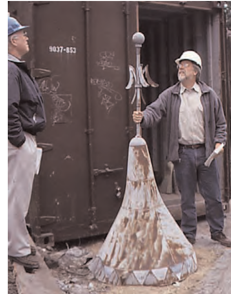
Architectural features that are in jeopardy of dislodging from buildings should be removed and temporarily stored until they can be permanently repaired.
