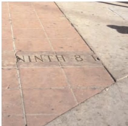
Terrazzo and inlaid bronze letters can be designed to indicate street names, orientation, and transit stops.
