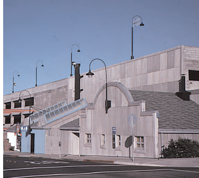
This parking structure near Cannery Row in Monterey takes into consideration the character of the historic canning facilities nearby. It fits into the overall historic context of the area. New structures in the Historic Downtown should strive to complement the historic building stock.
