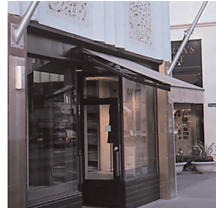
A single awning marks the entrance to this storefront, highlighting an inviting entry while leaving the storefront glazing with a larger area for displaying merchandise.
