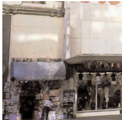
The main building entrances at either side of the Palace Theater are presently not evident due to the existing facade application. The above image shows a storefront located within one of the original openings.
