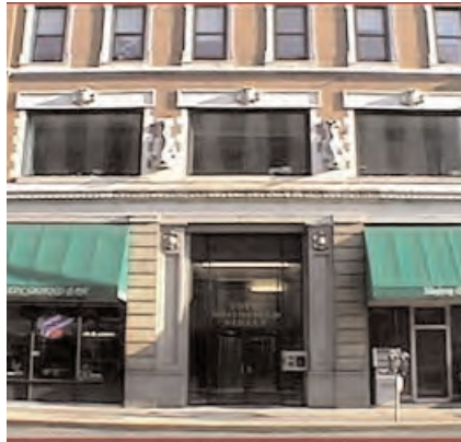
Awnings are a strong visual component of buildings and storefronts. These awnings are appropriately placed, but are somewhat too large for the storefront.
