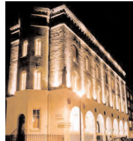
Before lighting the exterior of historic buildings, consider the building features to be highlighted. The building above is somewhat overly lit.
