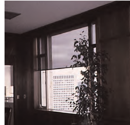
These interior shades can help with heating and cooling without affecting the character of the historic exterior.
