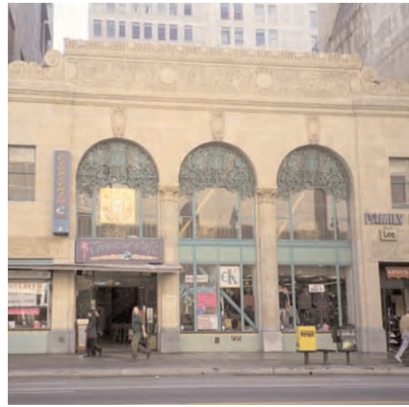
During rehabilitation the terra cotta facade was restored, the metal spandrels that divide the windows horizontally were uncovered, and limited and compatible signage was installed. Removing the metal awning would further reveal and highlight the building's decorative elements.
