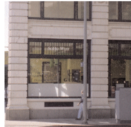
This storefront in the Apparel Mart Building is one of the few in the Historic Downtown that has remained relatively intact.
