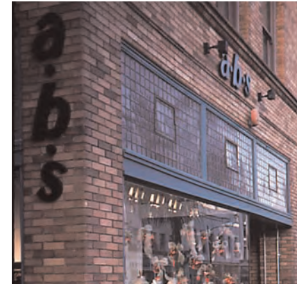
The "abs" sign on this store in Pasadena is made up of individual die cut letters that give a lightweight appearance to the sign.
