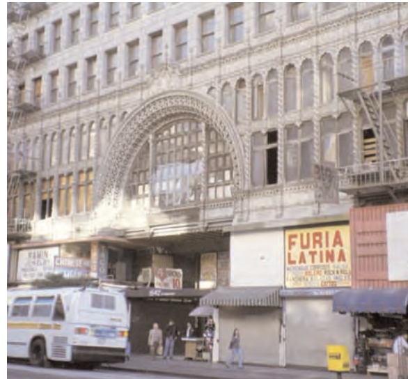
Today, the mezzanine level is completely lost under a layer of signage, and the storefronts have been removed and sub-divided. Reinstalling the glass at the mezzanine level will re-establish the building's original scale at the street level and heighten the connection between the interior of the building and the streetscape. Furthermore, increasing the transparency of the storefronts by re-introducing a glazing system, be it windows and/or doors, will likewise improve the building's street-level appearance, and restore its original vertical architectural divisions. Lastly, opening the mezzanine will allow more light into the upper stories of the building.
