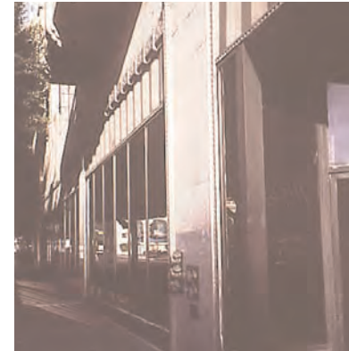
Setback: The absence of any setbacks usually describes an urban condition referred to as a street wall where continuous building facades align at the property line.
