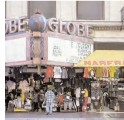
Typical of missing storefronts, the building elements that divide the store from the sidewalk are missing.
