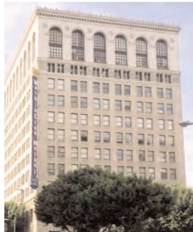
The middle stories of the Washington Mutual building have a distinct window pattern of two double-hung windows separated by a masonry spandrel. The corners are marked with a wider spandrel.
