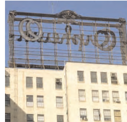
A rear view of the Orpheum Theater rooftop sign. When illuminated, this sign is visible at night throughout downtown.
