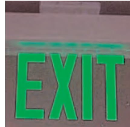
Clearly mark exits with appropriate signage.
