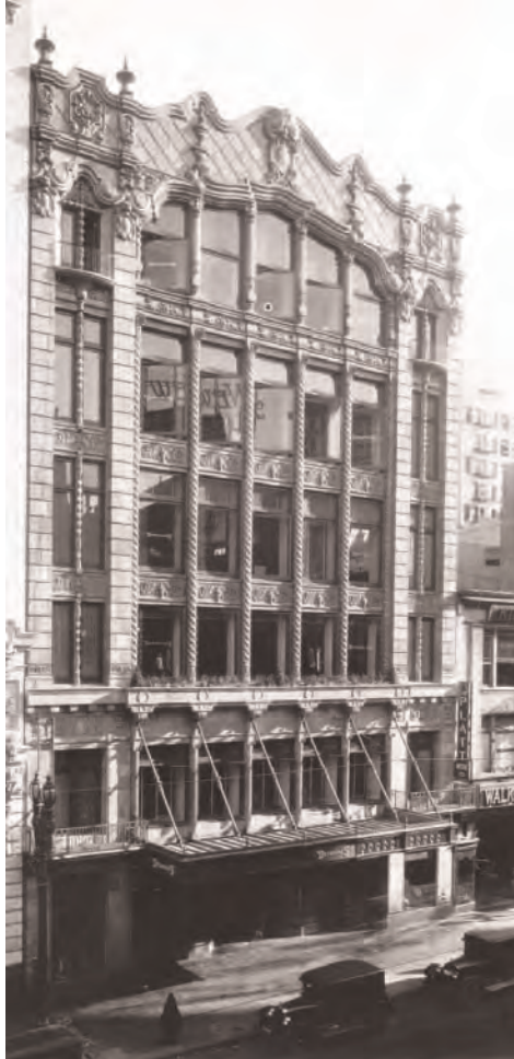
The Desmonds Store building located at 612 S. Broadway, constructed in 1924, has a polychrome terra cotta facade with twisted, engaged columns.
