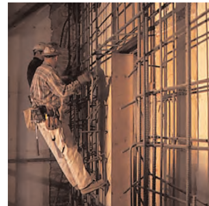
Shotcrete, spray-applied reinforced concrete, is another method of seismic strengthening.
