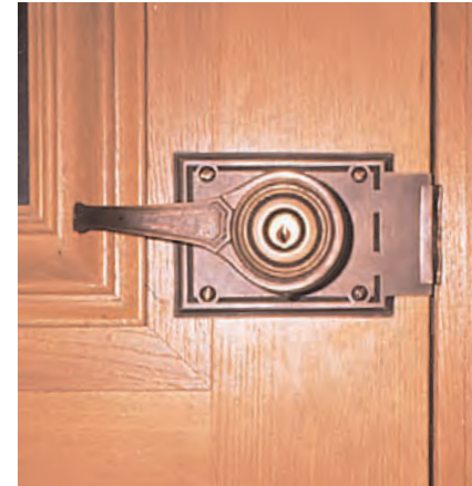
Historic door hardware can be modified to satisfy accessibility requirements.
