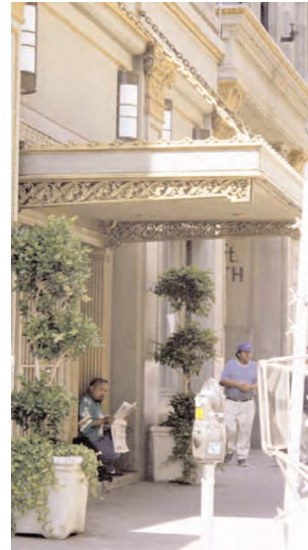
Metal and glass awnings are common throughout the study area and illustrate one use of metal as a building material. Proper cleaning and maintenance will ensure that metal awnings remain as one of the historic building components in the Historic Downtown.
