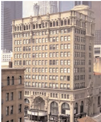
The heavy base of the Million Dollar Theater Building carries the structure with graceful arched openings into which are set the theater entrance and storefronts.
