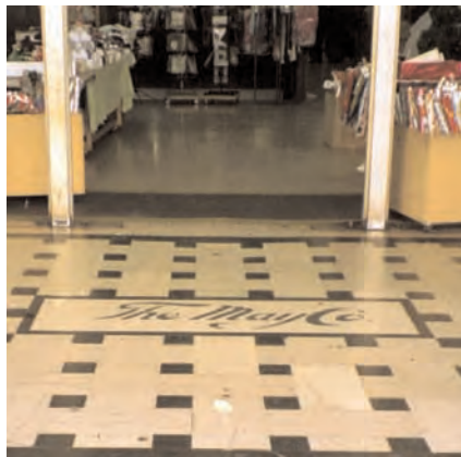
At an entry to the old May Company department store is an example of terrazzo patterning and inlaid signage. These examples of signage should be retained even when the original use or tenant no longer occupies the building.
