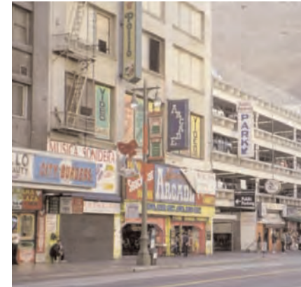
The removal of the storefronts has left the buildings with no scalable architectural features at the sidewalk.
