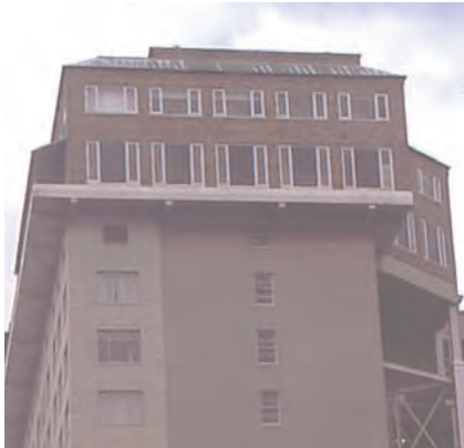
Rooftop additions can be problematic as there are frequently structural implications. This rooftop addition is not very successful in its design as it does not relate in fenestration pattern and is highly visible from the street.
