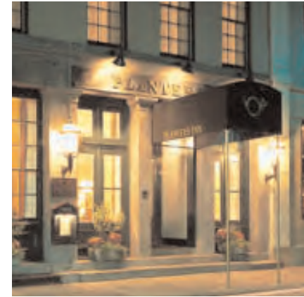
Accessibility is an important component of building rehabilitation. This historic hotel entry should be reconfigured to provide access.
