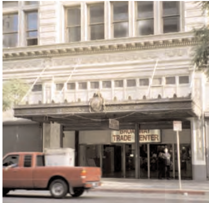
Lighting this entry awning at night should be considered. Either up lighting or pendant fixtures could be used.
