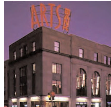
The 12-foot high illuminated letters atop the Philadelphia Arts Bank, a bank renovated to accommodate a rehearsal studio, draws attention from that city's busy Broad Street.
