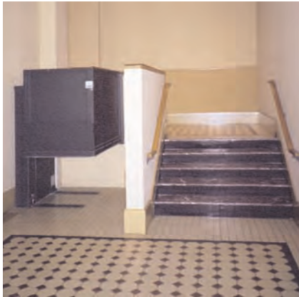
A handicapped lift can be useful where there is inadequate space for ramping. It should be placed in a non-historic space if possible.
