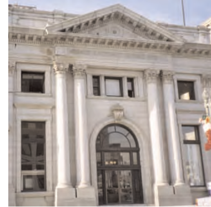
Cast stone is commonly used for very large building elements such as the columns on the historic Farmers & Merchants Bank.
