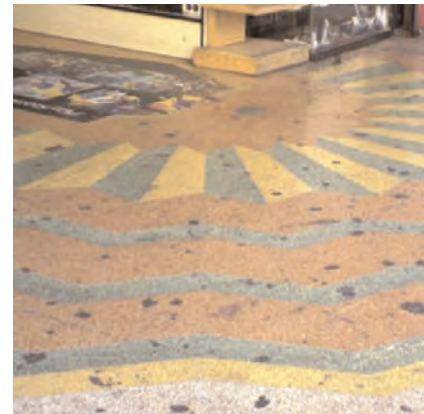
The terrazzo sunburst at the entry to the Arcade Theater.
