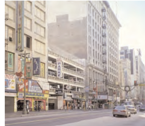
The non-contributing infill parking garage on this block breaks with the prevailing height, scale, and massing on the block. In the future, a taller structure, and with a more suitable fenestration pattern would be more appropriate.
