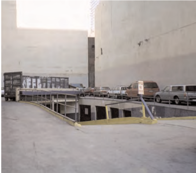
This entry to an underground garage encompasses an entire parcel. New parking structures should be designed with appropriate entries and features located at the street wall. Infill construction could occur on this lot in the future.
