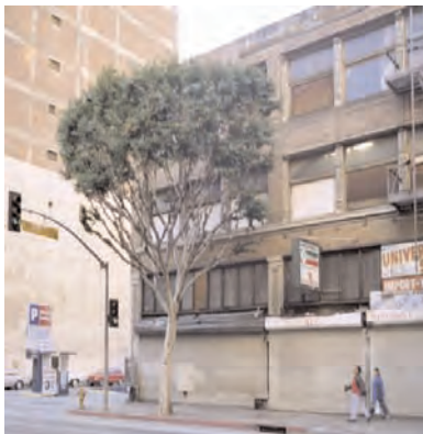
Transom Window: These windows are usually located above the storefront and below the sign area. In this case the roll down doors cover the storefront. Transom windows often are divided lights.
