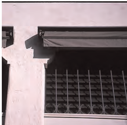
Retractable awnings such as these can help control heating and cooling of interior spaces, while allowing historic features to be seen.
