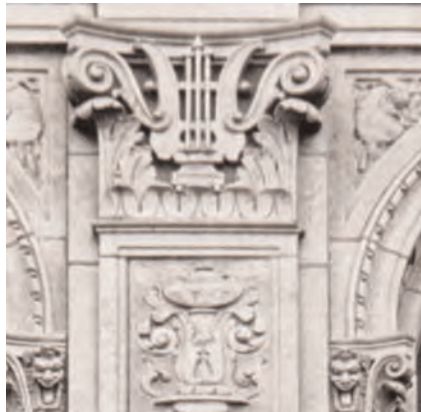
The Wurlitzer Building on Broadway is a virtuoso display of polychromatic and glazed terra-cotta ornamentation.
