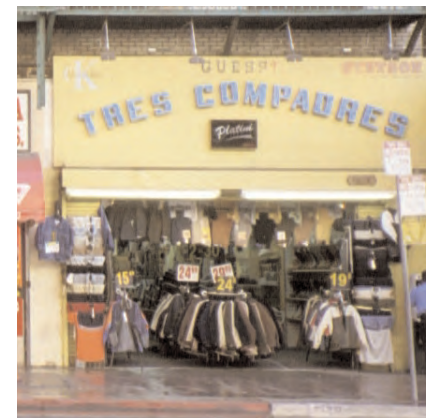
Some storefronts limit the display of goods to within the outline of the storefront. However, the lack of transparent glazing requires that a solid security door be used after shop hours.
