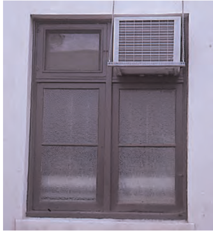
Window AC units are not very efficient and they detract from the appearance of the building.
