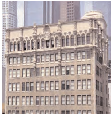
Replace in Kind: The upper story windows at the Million Dollar Theater are good examples of new features that replaced older windows with a similar type and style of window.
