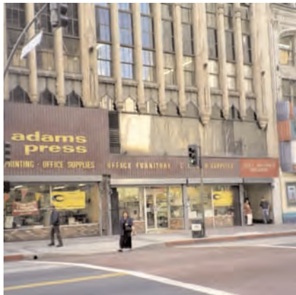
Wherever possible, the storefront should relate to the upper story elements. Here, as with many buildings, the transom has been covered.
