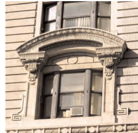
Simply cleaning and painting these wood windows would greatly improve the appearance of this building facade.
