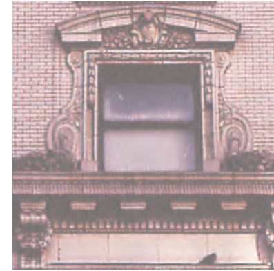
Dentils: These dentils on the Alexandria Hotel are located below the window and just below the modillions that are attached to the underside of the cornice.
