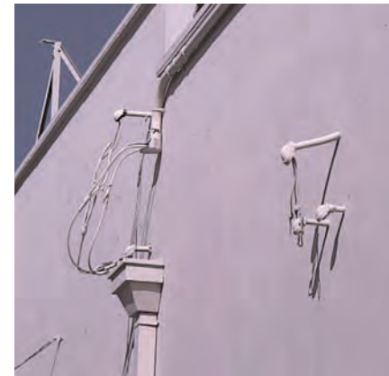
Most older buildings will require substantial upgrade of systems.
