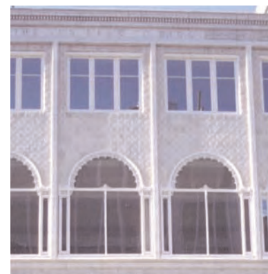
Bay: The Sun Drug Company building at Broadway and Sixth Streets employs bays to define the repetition of architectural elements.
