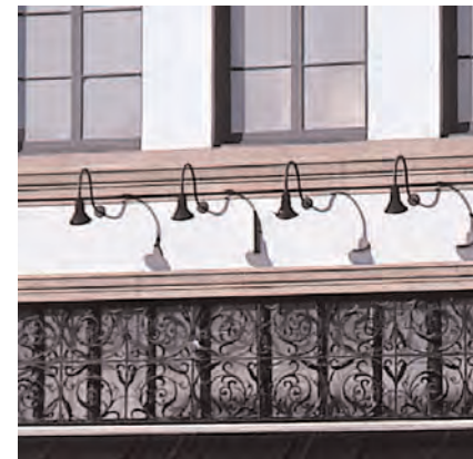
These gooseneck exterior wall-mounted fixtures cast light down onto the store's display glass and sign area.
