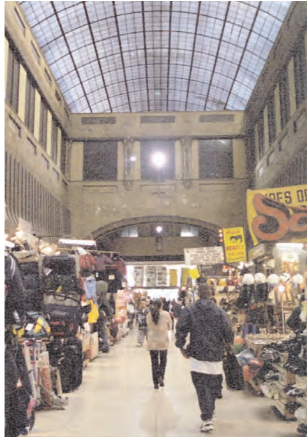
The arcade with its current configuration of merchandise display and signage. The screens at the lower mezzanine level and the removed glazing are apparent in this image.
