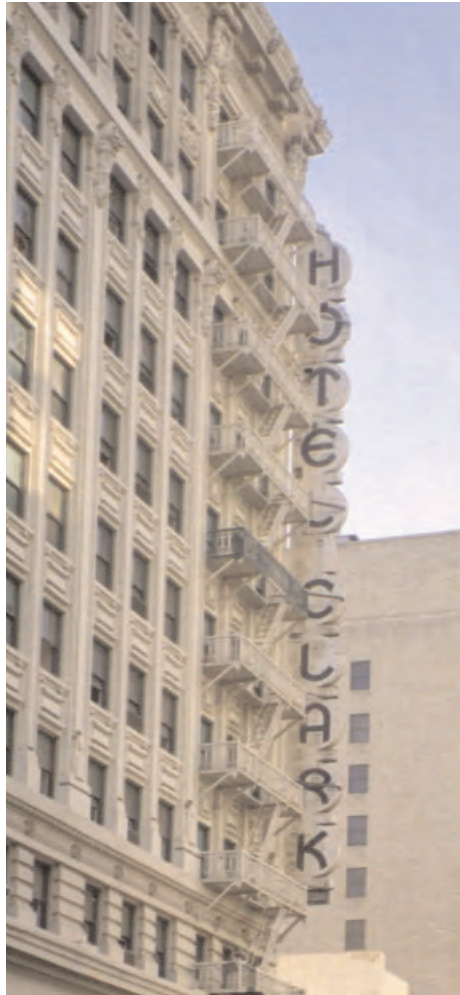
The terra cotta facade of the Hotel Clark are accented by both the metal fire escape and the metal vertical sign.
