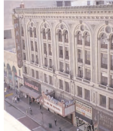
A view of the Palace Theater from across Broadway, showing the terra cotta detail at the upper floors and the alterations to the lower story.
