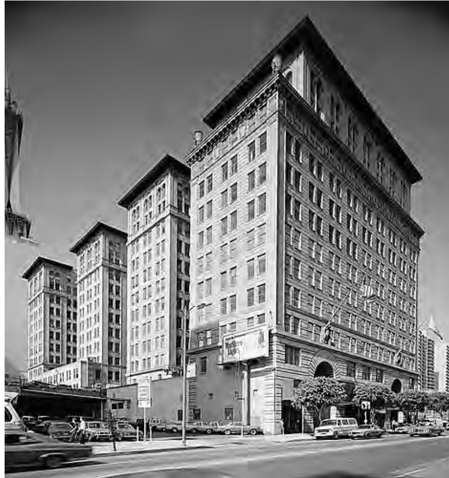
The Subway Terminal Building at 415 Hill Street circa 1980.
