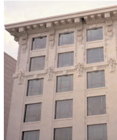
The top of this building has a heavy cornice that serves to terminate the verticality of the structure.
