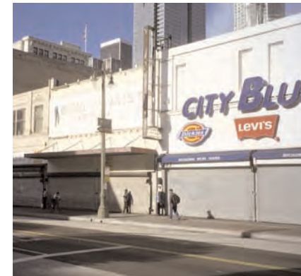
A similar view on Broadway underscores how a series of solid roll-down doors creates a very uninviting environment.
