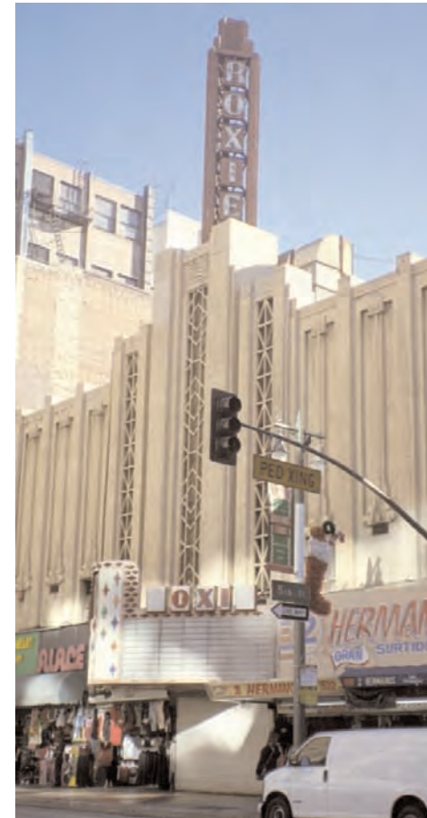
Some of the character-defining features of the Roxie Theater are its rooftop sign, the verticality of the facade, the location of the marquee, and the monochrome nature of the terra cotta.
