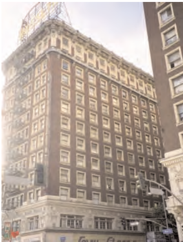
Historic Features: Some of the historic features of the Rosslyn Hotel are its roof and corner sign, windows, terra cotta elements, other masonry elements and the fire escape.
