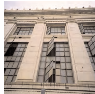
Pilaster: The pilasters on this building break up the window mass and help balance the horizontal and vertical character of the facade.
