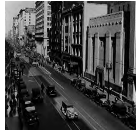
The Stock Exchange, built just before the market crashed, solidified Spring Street's position as the financial center of Southern California.
