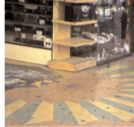
The terrazzo sidewalk outside the Arcade Theater. Note that the material spills out onto the sidewalk, unifying the indoor and outdoor space.
