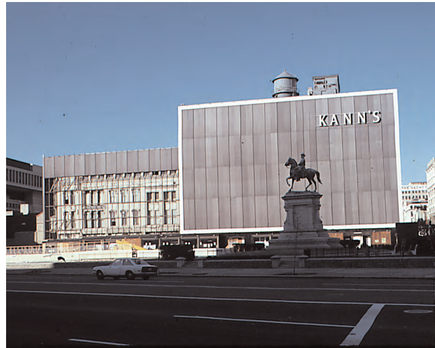
This department store in the midwest underwent facade rehabilitation. In this photograph, the historic building is visible on the left while the screen remains on the right.
