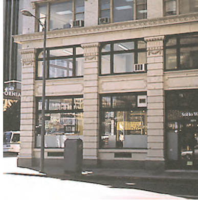
Plate Glass: Plate glass was used most often in commercial buildings with storefronts. Here the large expanses of glass highlight the storefront.
