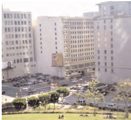
At the corner of Fourth and Hill there are two vacant lots across from Angels Flight park and the metro stop. Infill construction on these corner sites would re-establish the continuity of the street wall.
