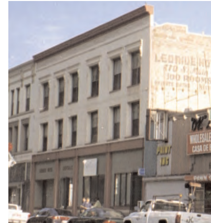
This building has a high parapet at the front facade that will serve to screen any rooftop mechanical equipment of a certain height.
