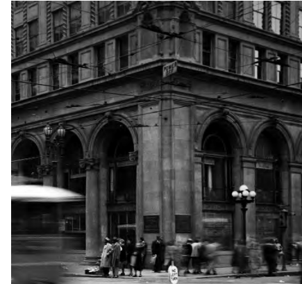
The grandness of Spring Street is conveyed through its monumental buildings.
