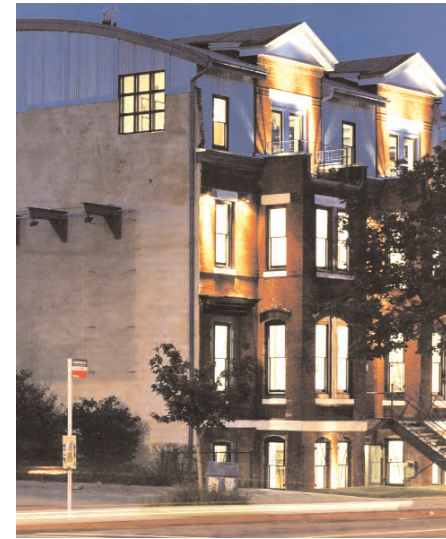
At derelict town houses in Washington D.C., a substantial amount of the original materials could not be salvaged. Therefore, new, more industrial materials were introduced where historic fabric was missing, and an addition was designed for the rear and roof of the original historic buildings.
