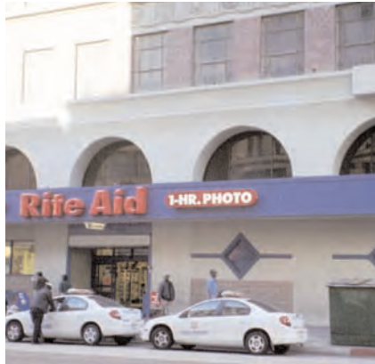
The character of this historic building has been altered by an inappropriate storefront remodel.
