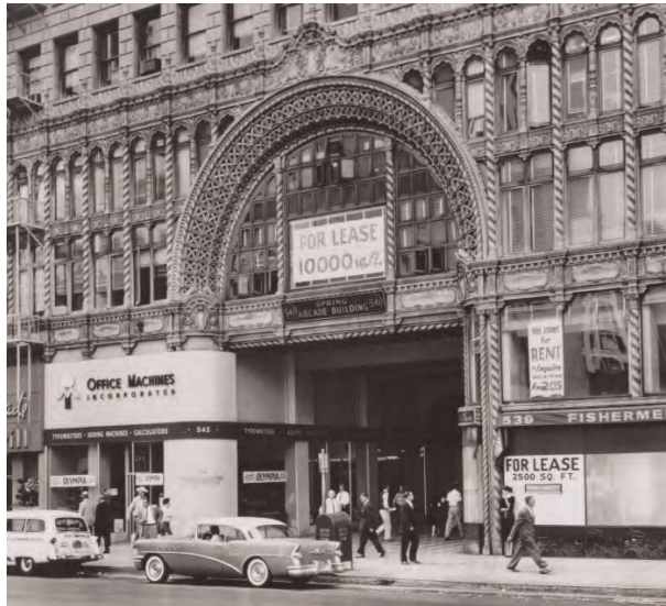
In the above image taken in the 1960s, the mezzanine glazing and original storefront configuration of the facade is still apparent. However, some facade alterations had occurred by the date of this photograph.
