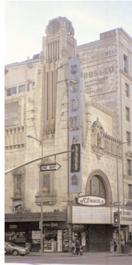
The prominent vertical, corner feature of the Tower Theater. This building has significant terra cotta decorative features that range in color and theme.
