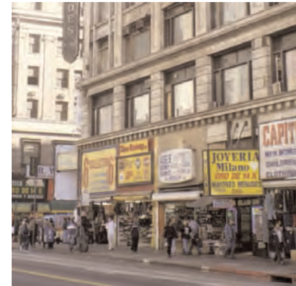
A typical commercial storefront building in the Historic Downtown, a multi-story building with commercial retail spaces at the street level.
