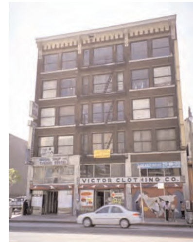
Frieze: The frieze accompanies the cornice to help define the building top.
