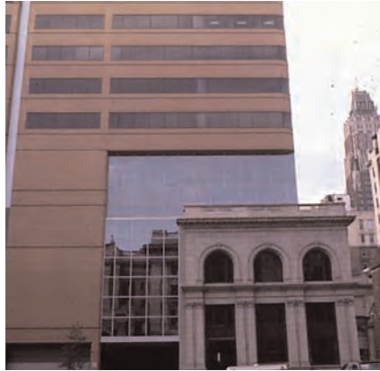
This historic bank building is engulfed by a high-rise addition. This type of treatment should be avoided.
