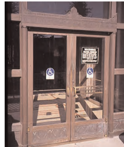
At this building, the designated accessible entry is clearly marked.
