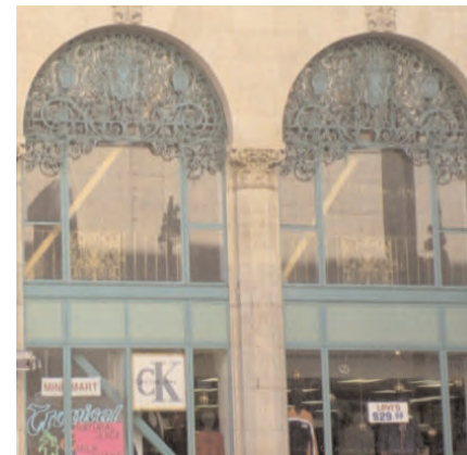
The Victor Dol Building incorporates metal windows and elaborate metal screens in the upper arches.
