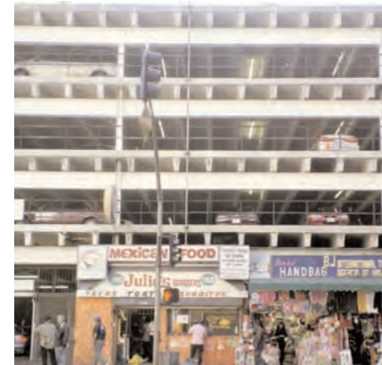
The parking structures on Broadway lend no interest or scalable features to the street and nothing to which pedestrians can respond. Some ideas for mitigating these features are illustrated on the next page.
