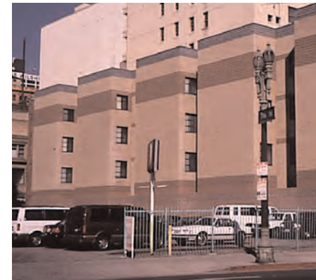
This infill construction between Main and Spring Street incorporates lightwells, anticipating a future building on the adjacent surface parking lot.
