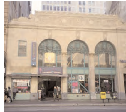
Most of the original architectural features of the Victor Dol Building facade have been retained and restored. Removing the awning over the entry would re-establish the vertical divisions of the building.
