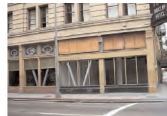
INTACT STOREFRONT TYPE
