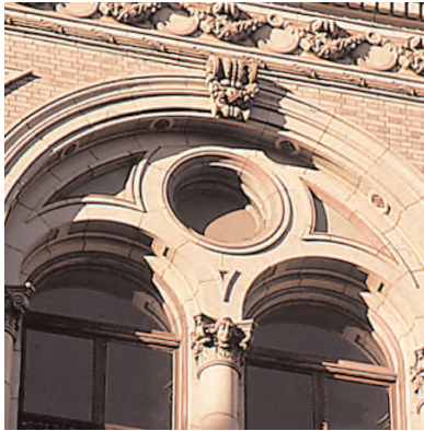
Keystone: In the case of this keystone on the Palace Theater, it is merely decorative rather than structural.
