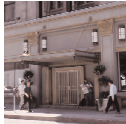
Another entrance to the same building. The building's original canopy is in place, color has been added to enhance and highlight architectural detailing, and lighting has been introduced.
