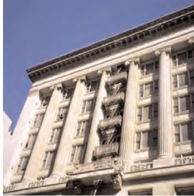
Capital: Ionic capitals decorate the tops of these columns, which carry a heavy cornice.
