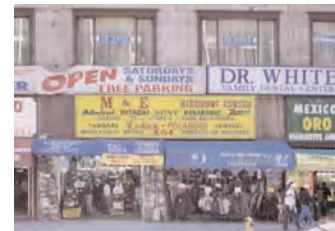
MISSING STOREFRONT TYPE
