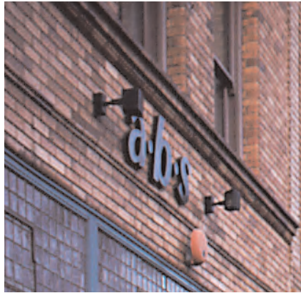
These light fixtures create a glow directly around the store's sign letters.
