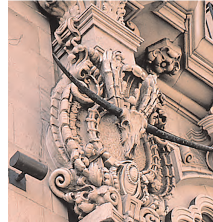
These decorative, terra cotta elements are character-defining features and should be retained and rehabilitated.
