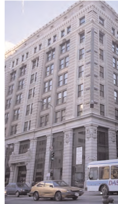
Existing masonry buildings with operable windows already function in an energy efficient manner. Making these windows operable again is an energy-conscious approach to cooling.
