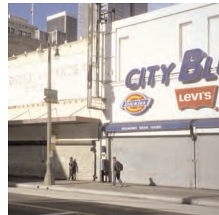
At the end of the business day, solid metal doors roll-down and seal the storefronts off from the street.
