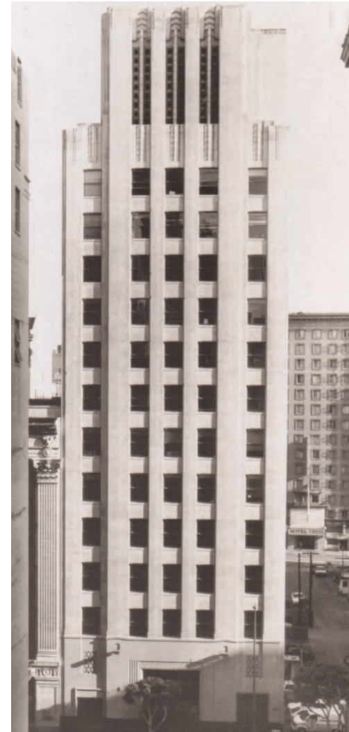
The top of the Banks Huntley building at 632 S. Spring Street. The upper facade is treated as a tower with vertical panels of chevron.
