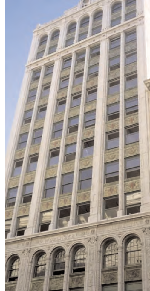
The Wurlitzer Building is typical of the buildings in the study area: it is a masonry- and terra cotta-clad structure. The above view shows the dramatic principal facade of this colorful building.
