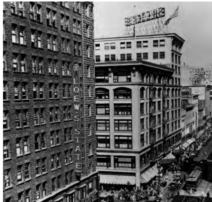
Although the width of the street has not changed, Broadway's sense of scale has increased with the removal of the rail lines.
