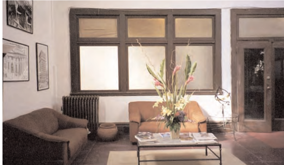
Above left is an image of a gutted office area, above right is an intact stairway and below is a rehabilitated office space at the upper floors of the Palace Theater. The remodeled office project retained the historic door; interior windows to the hall, and the historic radiator. An open, airy quality is achieved.
