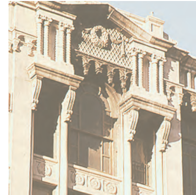
Mullion: Mullions are the vertical members between adjacent window sash or panes.
