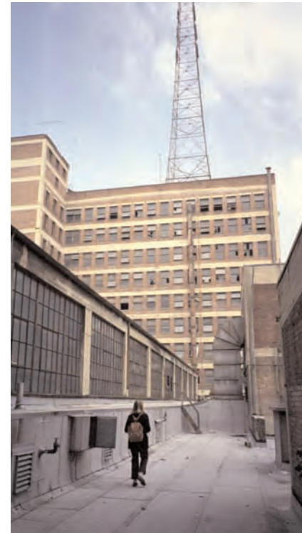
The rooftop above the arcade that connects the two towers. This area would be conducive to new rooftop uses such as a small community garden for residential tenants or as an outdoor gathering area for office workers.
