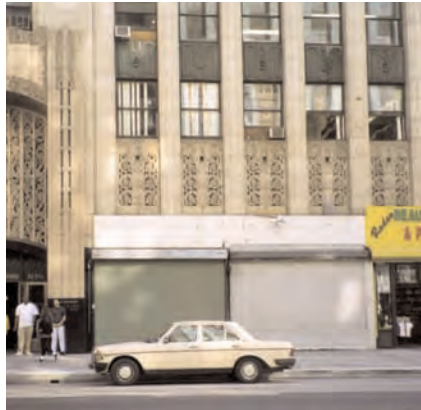
Roll down doors are one of the major intrusions within the study area. These features cover and detract from the historic components of storefronts.
