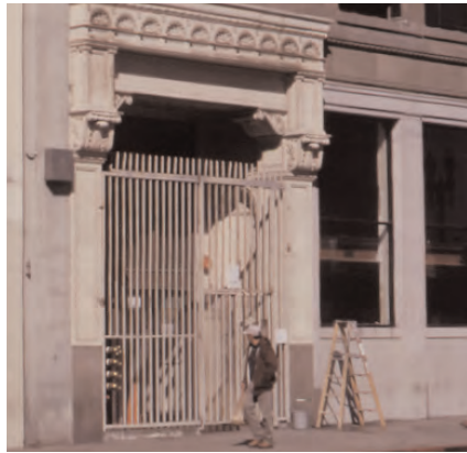
Before the side entrance to this building was rehabilitated, the security gate yielded an uninviting space.
