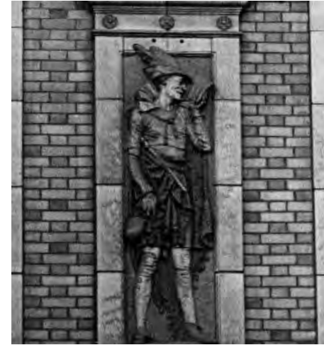
A detail of a harlequin on the Orpheum (now Palace) Theater at 630 S. Broadway. This theater, constructed in 1911, made use of multi-colored terra cotta on the facade.
