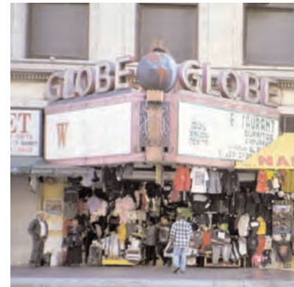
Do not infill recessed theater entrances when building use changes. The shop should utilize the interior of the building and leave the entrance open as a store-front entrance area.
