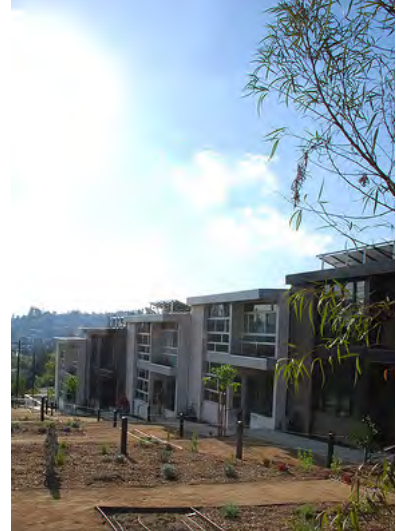
The Auburn 7 development provides enhanced landscaping along a DWP easement as a unique amenity for its residents.
