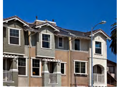
The Gatsby Homes in Hollywood demonstrates how to use different materials in response to building mass.
