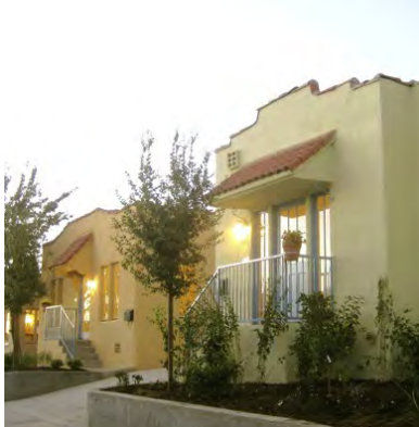
Small overhangs above the doors at Maltman Bungalows provide shade and shelter, as well as adding articulation to the entryway.
