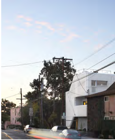
The Buzz Court development alternates texture, color, and materials on the front facade.
