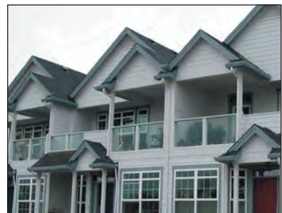
Excessively varied and multi-pitched roofs risk create visual chaos.
