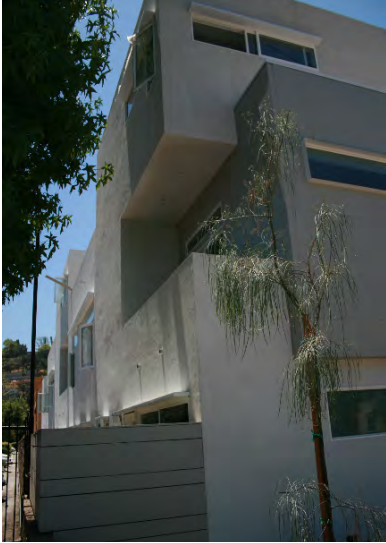
Sensitive window and balcony placement in the Rock Row development are key to enhancing the light and ventilation of the home's interior.
