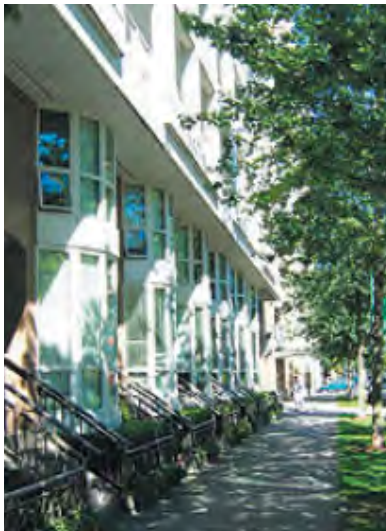
These home entrances sit a few steps above the sidewalk. A small landscaped area provides a buffer between the sidewalk and building edge.
