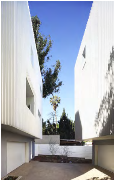
Small lot homes must be structurally independent with no shared foundations or common walls.
