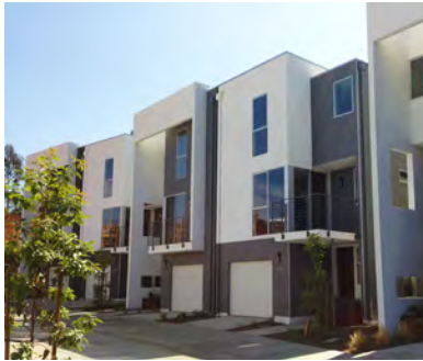
The Small Lot Ordinance allows for subdivisions in areas zoned for multi-family or commercial uses, permitting the development of this small lot in Echo Park.
