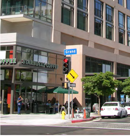
Corner curb extension at Grand Avenue and 11th Street.
