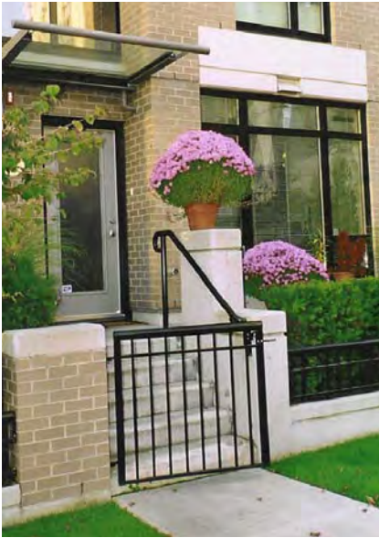
Good example of individual unit entry several feet above the sidewalk with porch and windows that look onto the street.
