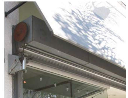
Awnings can be used to conceal existing exterior roll-down doors during business hours. Left: overall view of the storefront. Right: detail of the grill housing.
