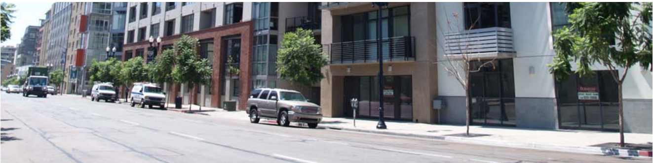
Good example of horizontal variation along a façade.
