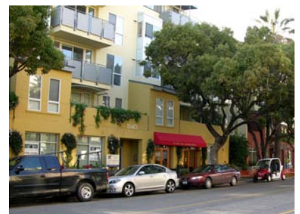
Good examples of an identifiable break between ground level retail and the upper floors.
