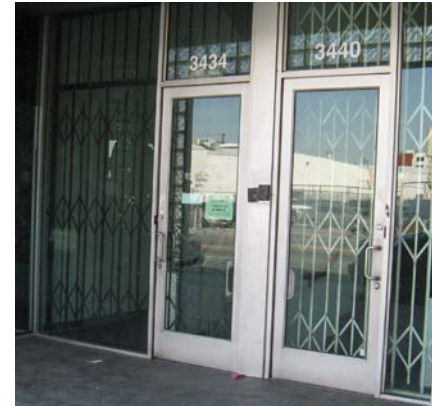
Interior grilles that are more than 75% open are less visible during non-business hours and easier to screen from view during business hours.
