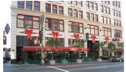
Good examples of buildings that promote sidewalk activity with overhangs, awnings and other transitional elements integrated into the architecture.
