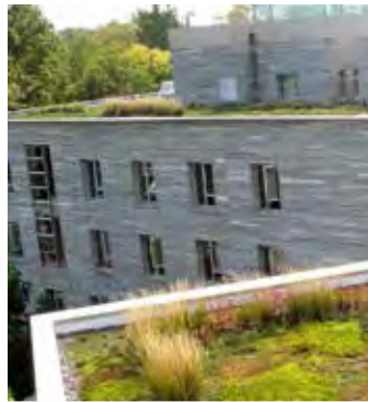
Green roofs help minimize stormwater impacts from storms {Philadelphia, PA}
