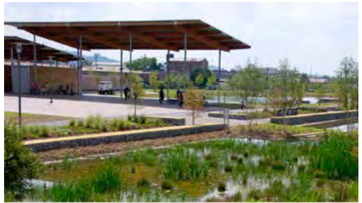
Engineered wetlands treat wastewater and runoff before reintroduction into the water system {Birmingham, AL}
