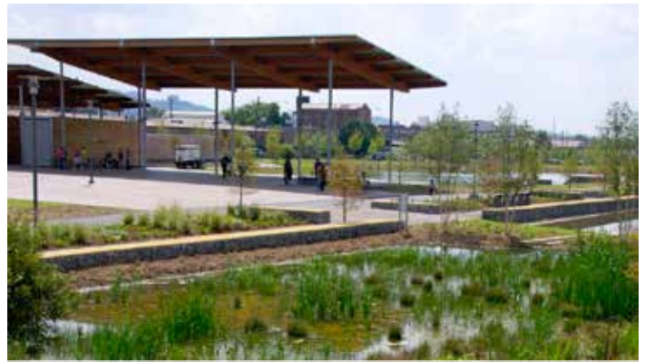
Engineered wetlands treat wastewater and runoff before reintroduction into the water system {Birmingham, AL}
